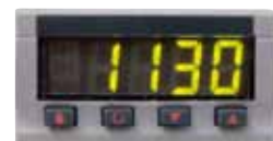
Over-temperature limit controller
