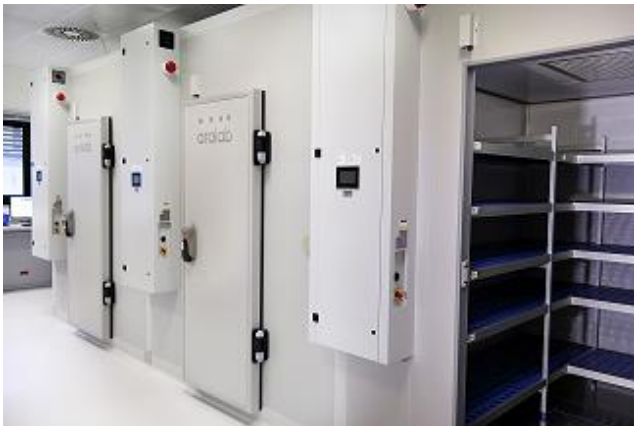
Stability rooms turnkey project by Aralab
