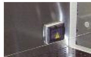
STANDARD ALUMINIUM NIGHT-DOOR PANEL AND ELECTRICAL OUTLET
